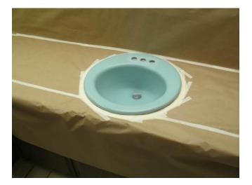
The surface is sanded and repaired with a durable filler. The area is masked and prepared for surface application. Other areas in bathroom are covered.
