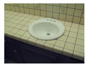
The masking material is removed and the surface is allowed to cure for an additional 24 hours. After this period the enclosure and hardware are replaced and ready to use.
