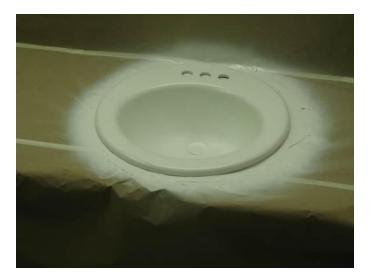
High volume temporary <u>ventilation</u> system is installed in the bathroom to prevent any chemicals from entering living spaces. The coating material is applied and allowed to set.
